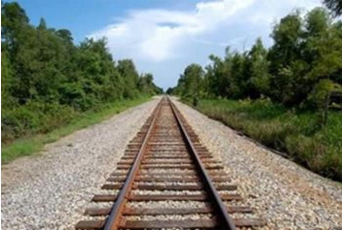
The U.S. Standard Railroad Gauge (distance between the rails) is 4 feet, 8.5 inches. That's an exceedingly odd number. Why was that gauge used? Because that's the way they built them in England, and English expatriates designed the U.S. Railroads.
