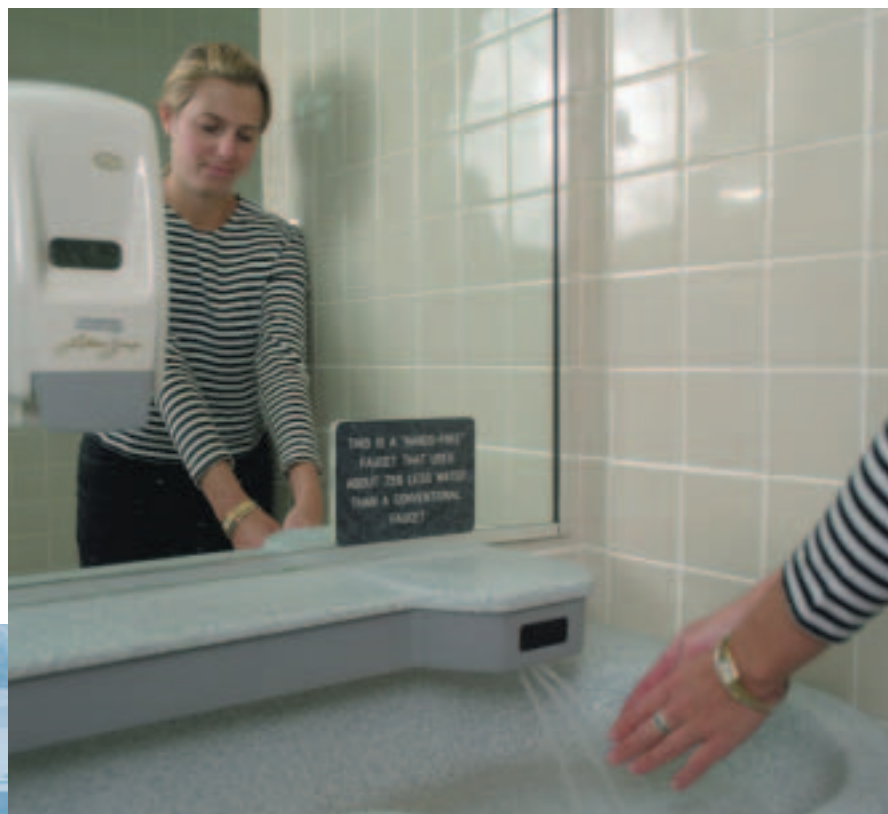
Sensors that automatically shut off faucets and flush toilets improve hygiene, comply with Americans with Disabilities Act (ADA) requirements, and save water.
