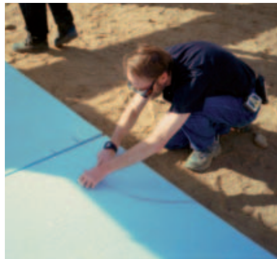
Installing rigid insulation under a floor slab minimizes conductive losses to the ground. Ground losses in well-designed buildings without slab insulation can be the greatest source of heat loss in these buildings.
