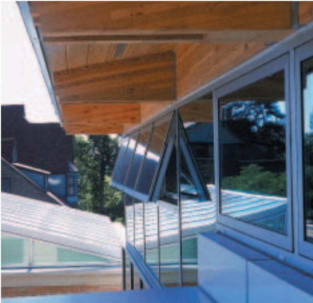
Operable clerestory windows automatically open when natural ventilation is appropriate for cooling the Lewis Center for Environmental Studies at Oberlin College in Oberlin, Ohio.
