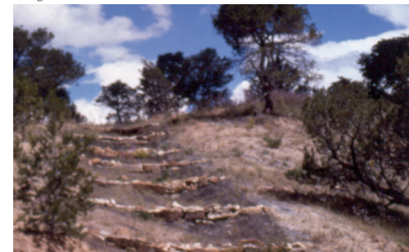
Image IV-3: Erosion Control - Check Dams
